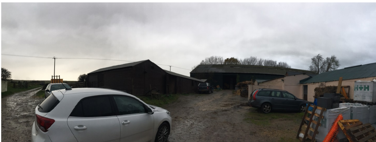
Photo 1: View of part of site looking North West
